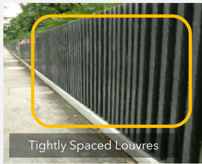
Figure 3.6 - Pedestrian access with Tightly Spaced Louvres
