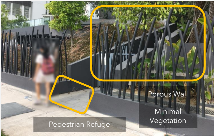
Figure 3.4 - Pedestrian Access with Porous Wall and Minimal Vegetation
